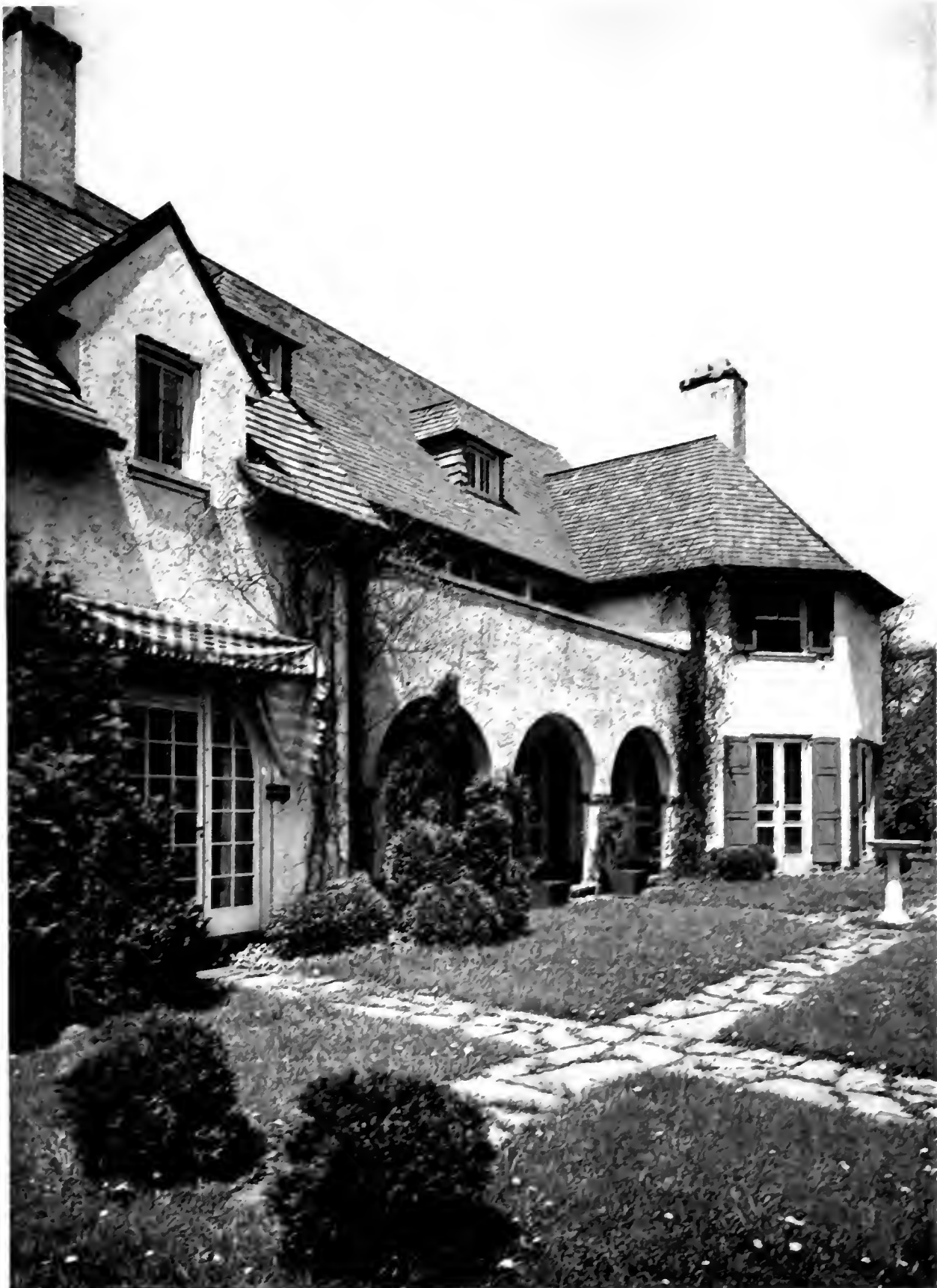
HOUSE OF MR. NORMAN MACKIE, CHESTNUT HILL, PA. ROBERT R. MCGOODWIN, ARCHITECT
